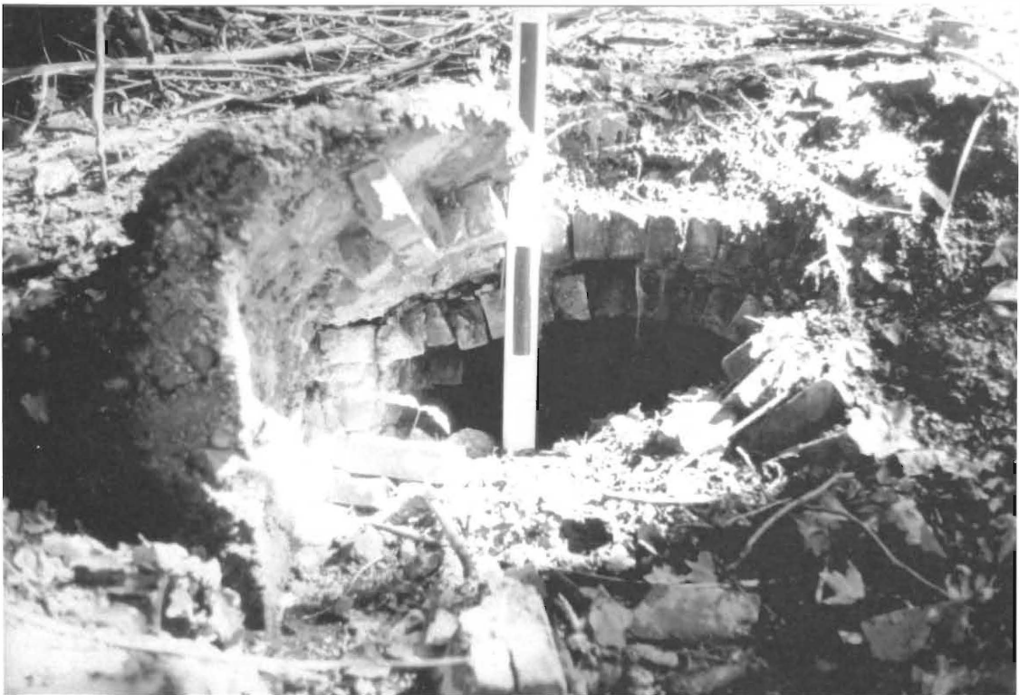
Photo 10. View east of a below-ground race on the northern right-of-way line that carried water from the upper factory complex to the lower factory complex.
