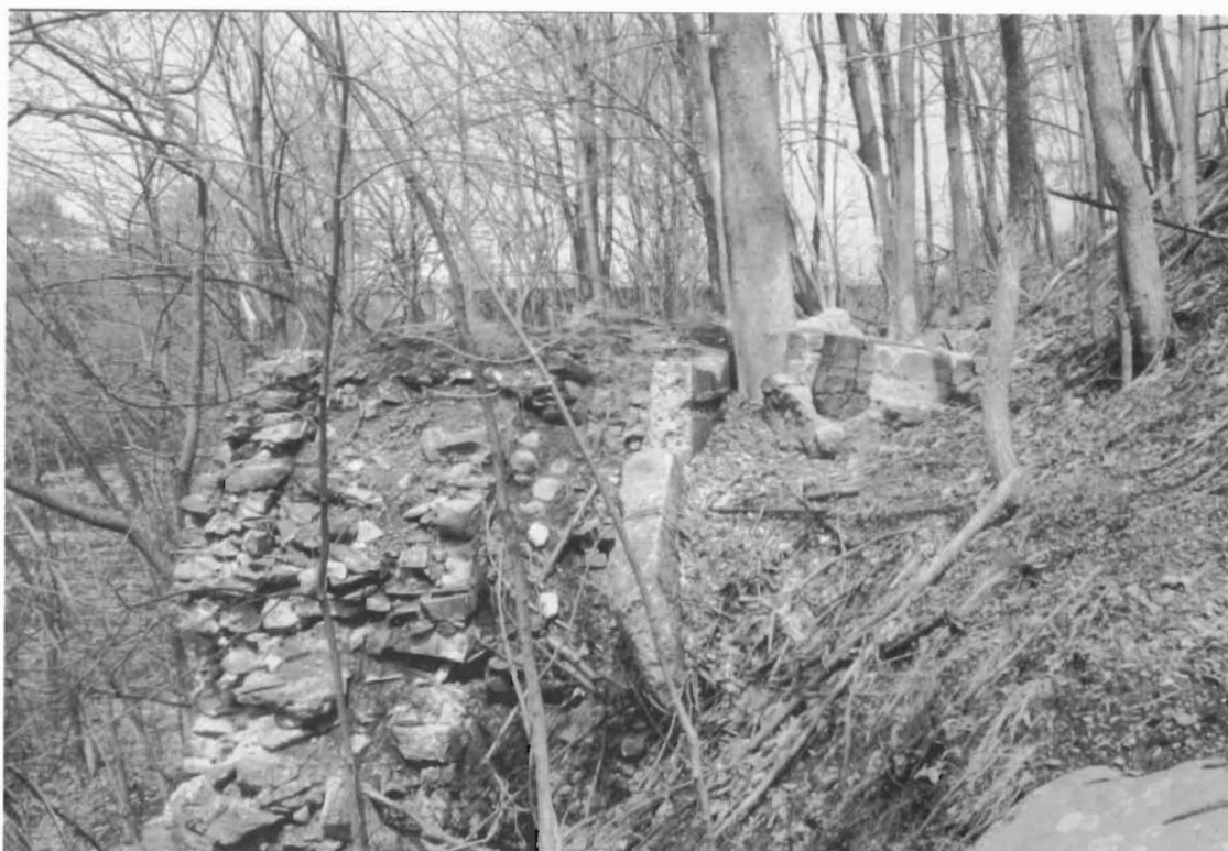
Photo 17. View south of the upper mill race on the right side of the photo. The mill race ran through the east end of the original six-story factory building and the carpenter shop.
