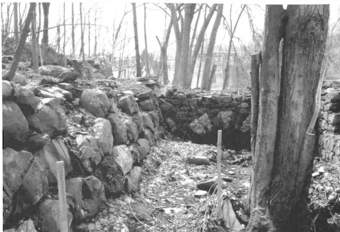
Photo 20. View south of the stone-arch – covered tailrace (Feature 5) with Units 1 and 6 located on top of the arch in the center of the photo. The stadia rod is in the race.
