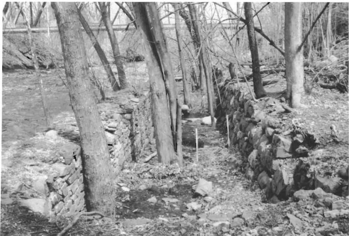
Photo 4. View north of the project area of the north wall of the building foundation and mill race located in the project area. The stake in the center of the photo is the centerline and the stake on the right, or east, is the right of way marker.
