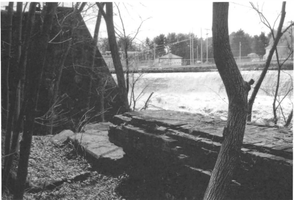
Photo 18. View southeast of the modern Niagara Mohawk power dam located adjacent to the south side of the original 6-story factory building. The construction of the current dam impacted the location of the original headrace and dam.
