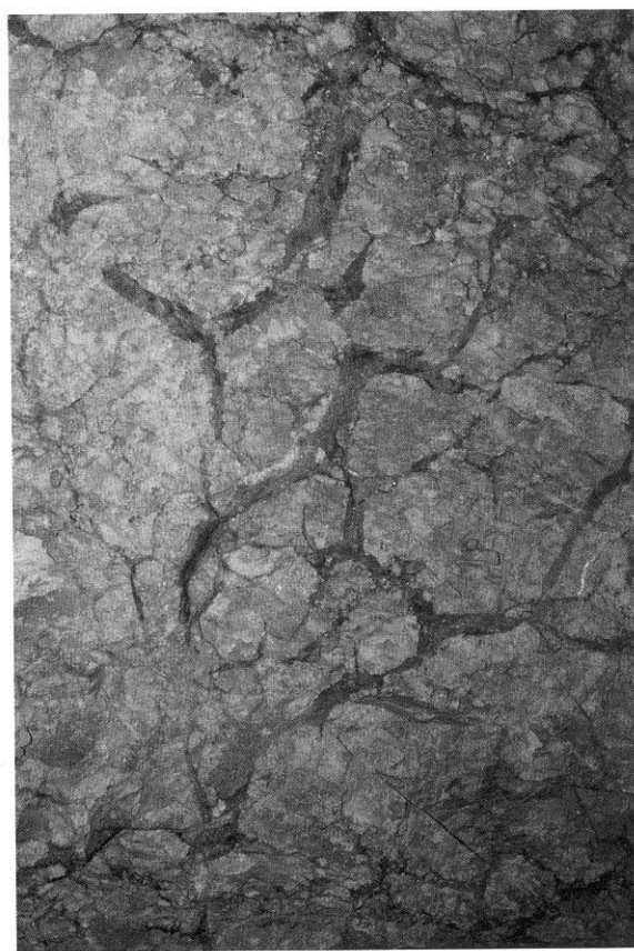
Photograph 4: Roof of Retsof Mine where the B-6 salt had fallen away, revealing a polygonal network of reddish-orange salt-filled fractures.
