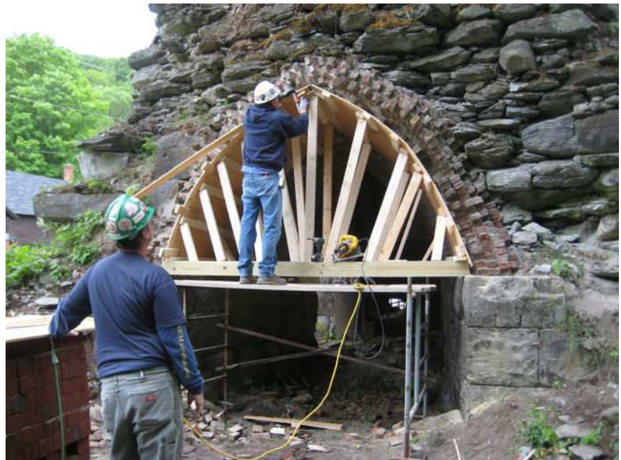
Figure 6.5. A June 2013 image of masons stabilizing the eastern arch of the furnace stack. The masons are using a combination of new brick for stability and collected older bricks from the arches for the exterior areas visible to the public. Image contributed by Friends of Taconic State Park.
