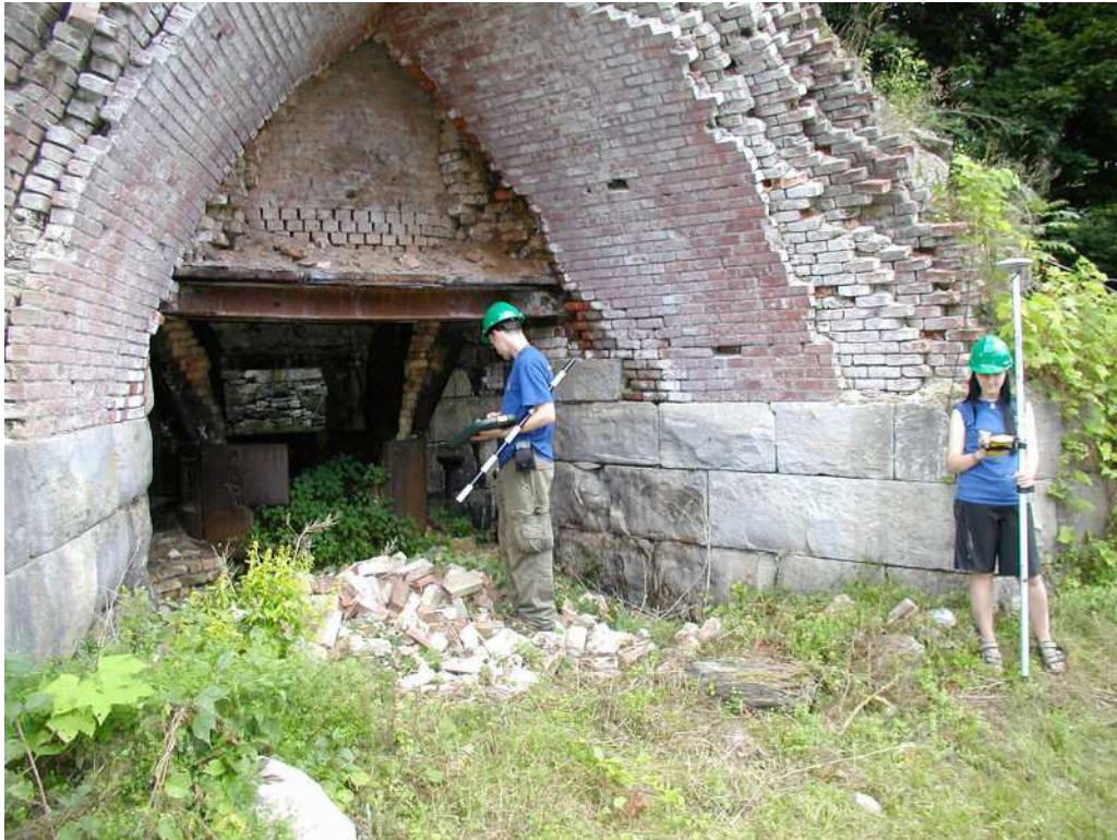
Figure 6.7. The author recording physical details of the furnace stack with assistant Sarah Rehrer collecting GPS point data in 2007.
