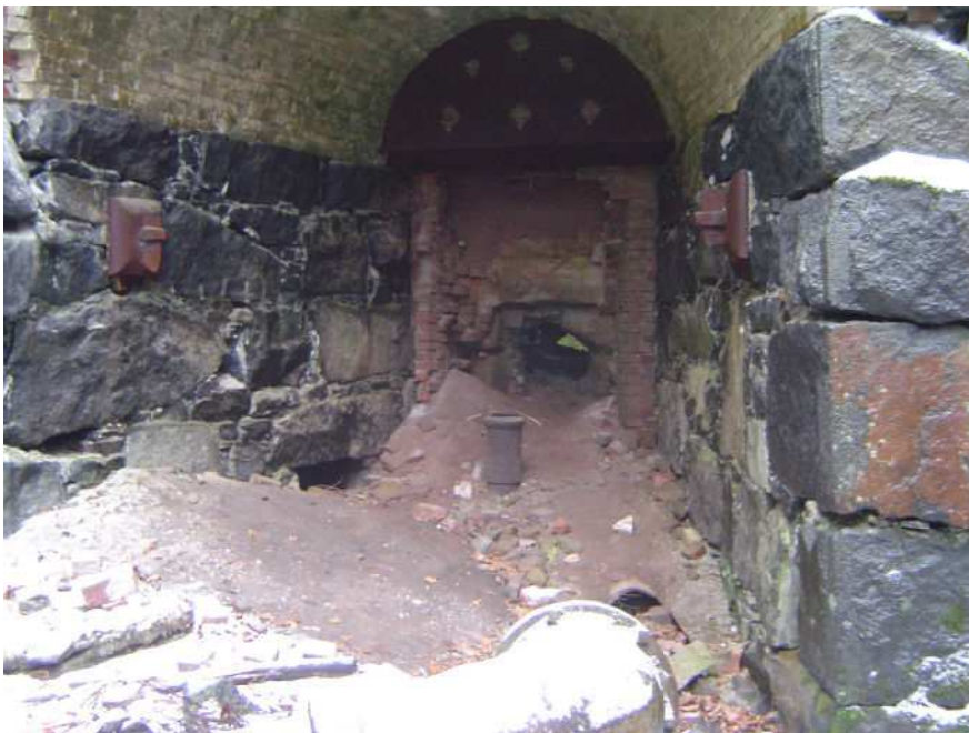
Figure 7.18. Southern arch (Photo Charles Vandrei, DEC 2003). Now much of the brick face is gone and the irregular arch surface is covered with fine soils.
