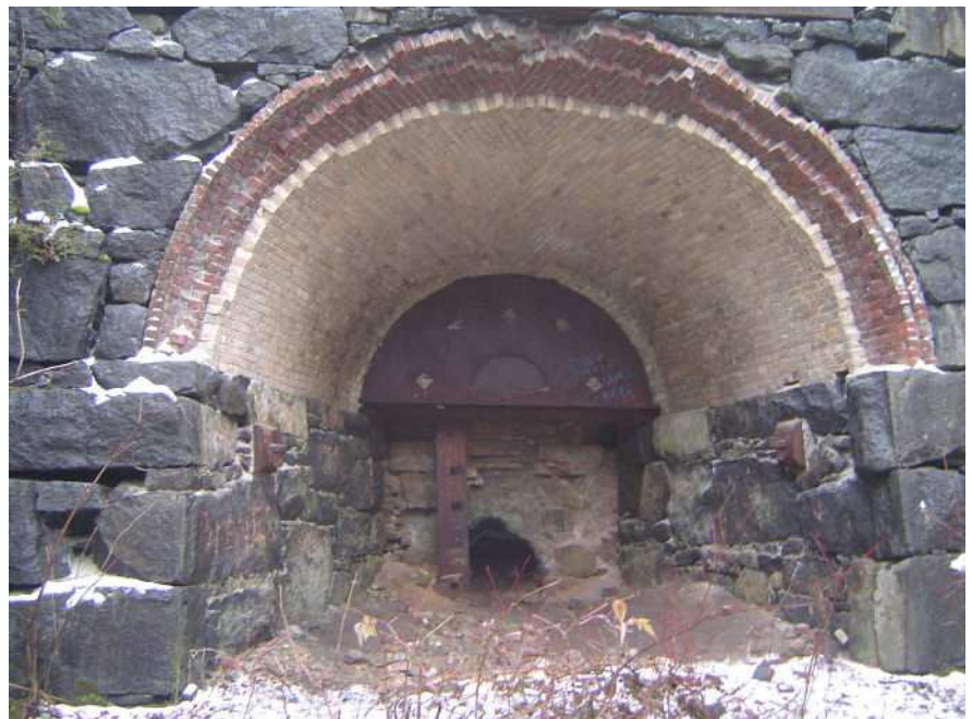
Figure 7.16. Eastern arch (Photo Charles Vandrei, DEC 2003). Twenty five years later the arch face is deteriorated, buckstay missing, and the soils are banked against the side walls.
