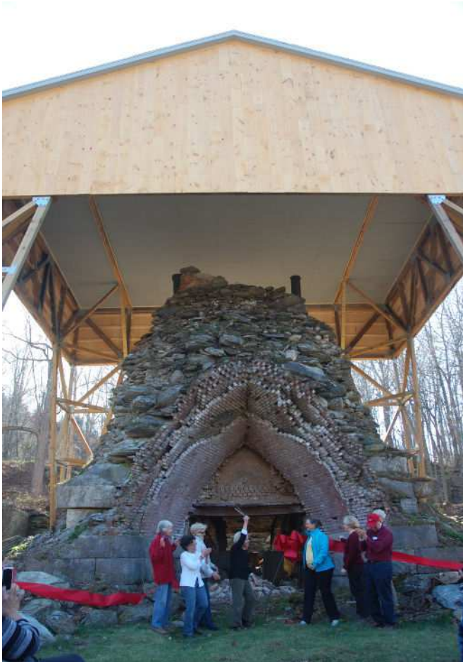
Figure 6.4. A recent (2013) image of the of the 1872 Copake Furnace stack with a new cover being dedicated by Friends of Taconic State Park board members. Note the lack of casing stones above the courses of marble along the bottom. This situation has led to extensive erosion of the brick and stone interior of the furnace since the late 1920s. Further stabilization should allow the stack to survive for another generation to appreciate. Image contributed by Friends of Taconic State Park.
