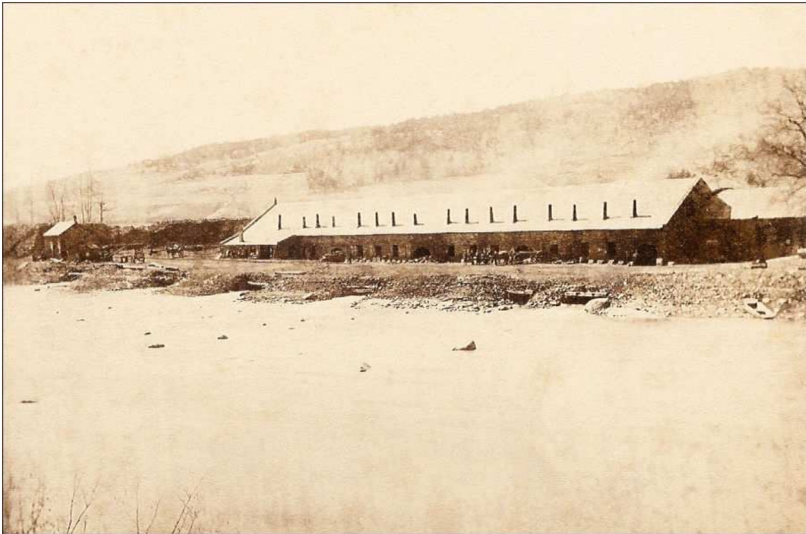
Figure 1.34. PS&I Co. stone forge with sixteen bloomery forge fires, looking northwest. G.W. Baldwin stereoview 1876. Collection of Gordon Pollard.
