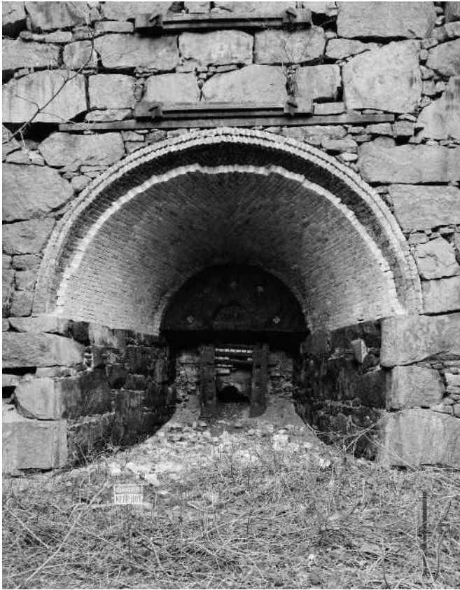
Figure 7.15. Eastern arch (Photo Jet Lowe HAER 1978 ). Photo shows the condition of the site in 1978 with both buckstays in place, vertical crossbars and bricks intact, and the general configuration of the ground surface in the arch.
